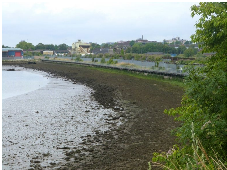
Figure 20 - Boardwalk in Southampton
